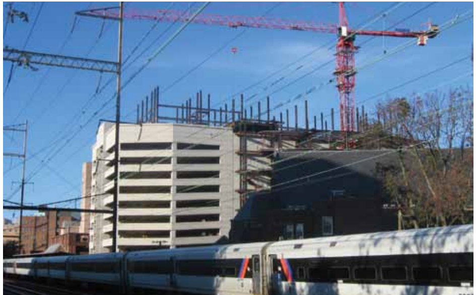
Erection of Steel Residential Tower over Precast Garage.
