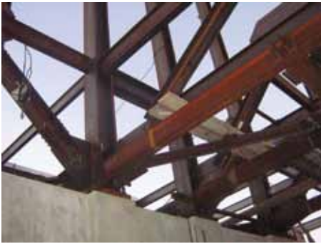
Steel Column and Brace Supported by Precast Garage Wall.
