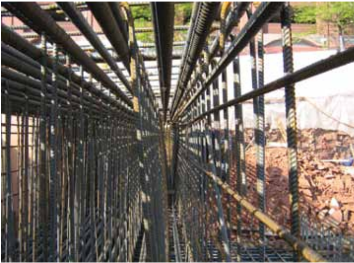
Deep Cast-In-Place Footings and Tie Beams to Resist Overturning at the Base of the Precast Walls.
