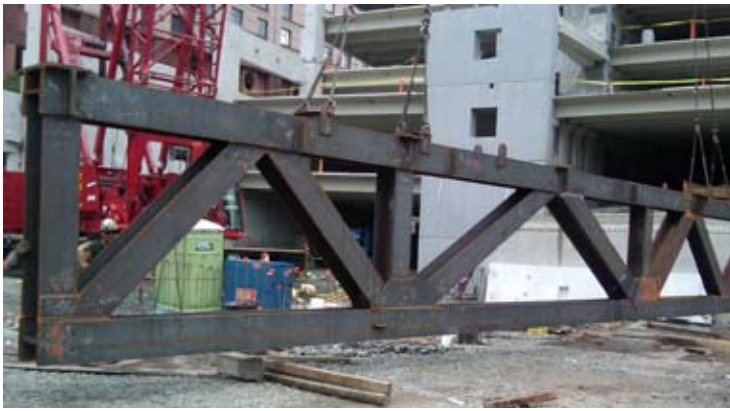
◀ Erection of a steel transfer truss.
